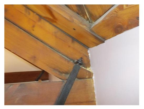
4) Approximately eight inch by two inch by two inch area of decay on the bottom edge and face of then diagonal chord
