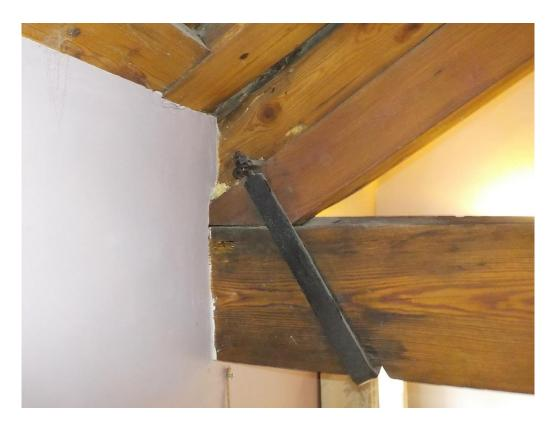
3) Approximately 6 inch by two inch area of decay appearing black along the top of the diagonal spacer.
