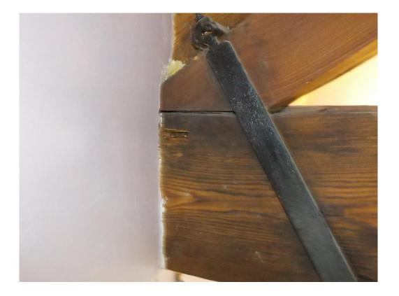
2) Approximately two inch by three inch area of decay on the horizontal chord immediately adjacent to the face of the wall.
